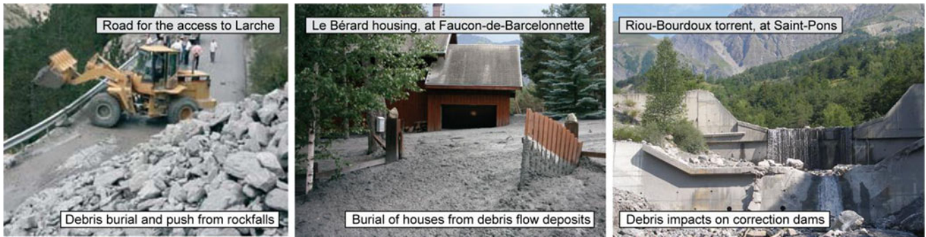
Fig. 3 Example of damage and consequence of several landslide types on categories of EaR observed in the study area in the last decade
